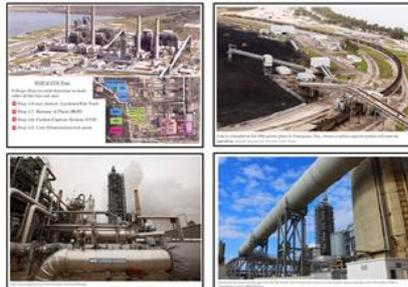
A 240 MW carbon capture system (CCS) processing flue gas from a subcritical oil of WA Parish Unit 8 to capture approximately 1.6 million tons of CO<sub>2</sub> annually that will be used for enhanced oil recovery (EOR) operations on the Texas Gulf Coast beginning with the West Ranch field in 2016
